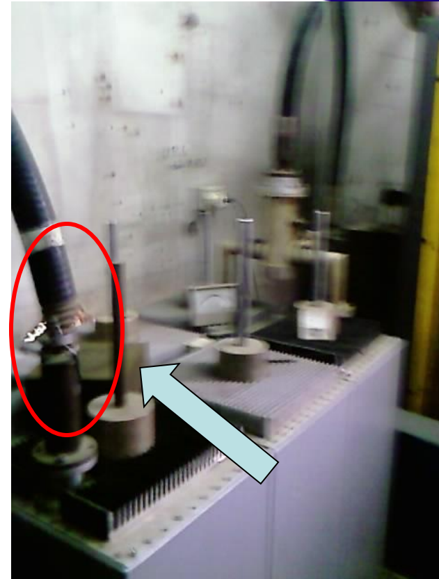
Bad Connector out from FM transmitter
